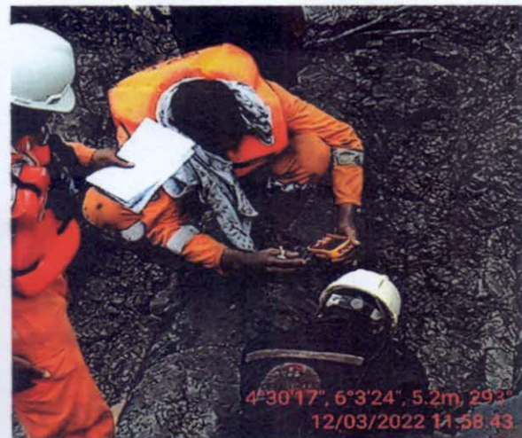
FIG. 1: SHOWING UTM TEST BEING DONE ON THE PIPELINE.
